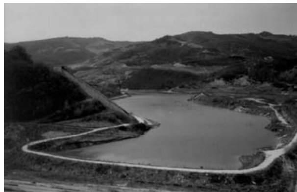
Figure 2. Reservoir: partial filling in spring.
